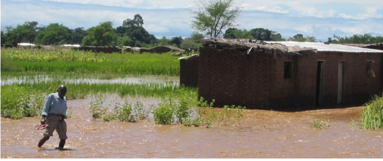
PHOTO 1 Houses in floodwater-holding zone during flooding
